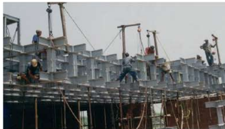
Figure 14: Manual module erection, the next sitting on the previous
