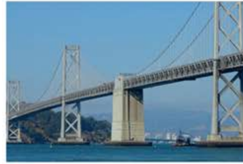
(b) San Francisco Oakland Bay bridge: Mid anchorage system
