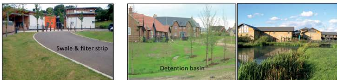
Figure 3: Components of SuDS (Environment Agency, 2018)
