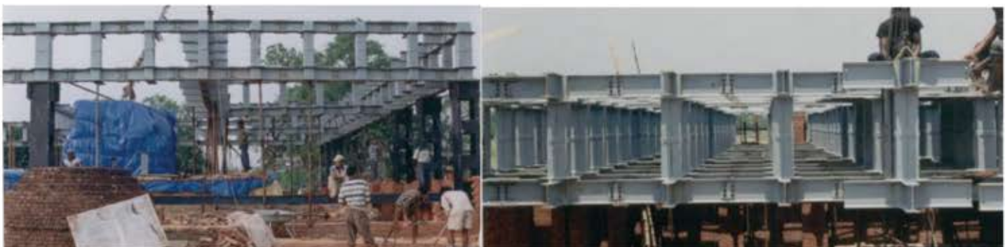
Figure 12: Beam Module Grids and General modules in between
