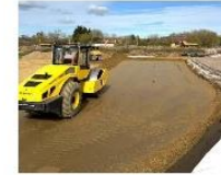
9J1 for UEF embankment
