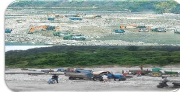
Figure (2) : Existing practices of Local river sand/gravel extraction/ mining
