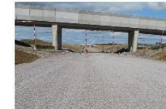
6F8 for sub-grade filling
