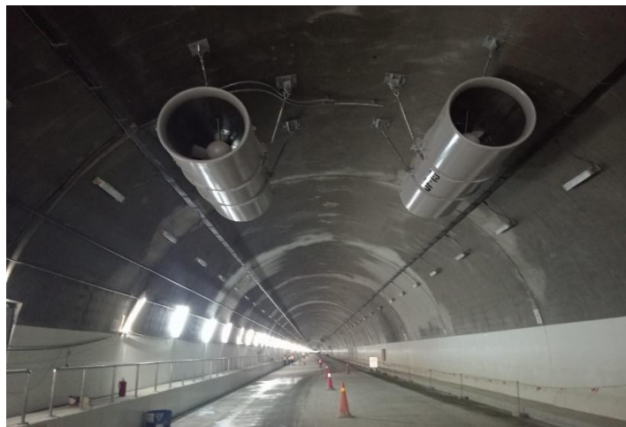
Figure 3: Installation of Jet Fan at Nagdhunga Tunnel Construction Project (Source: - NTCP Project, HAC-Kandenko-subcon)
