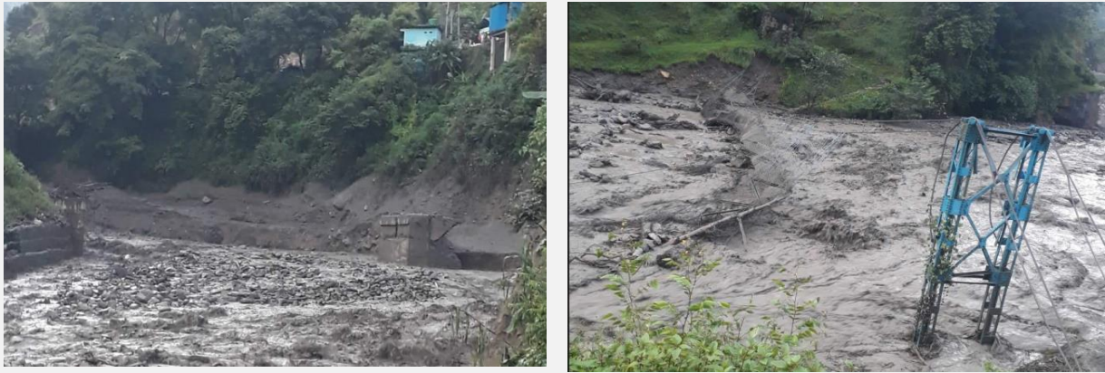
Figure 6: Laskugad Bridge along Mahakali Corridor after flood dated 9 th Sept, 2022
