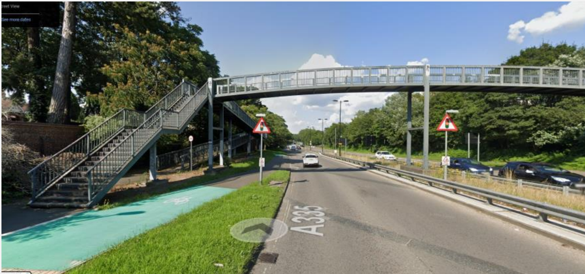
Figure 3: Pedestrian footbridge with ramps in Southampton, UK (Source: Googlemap, 2023)
