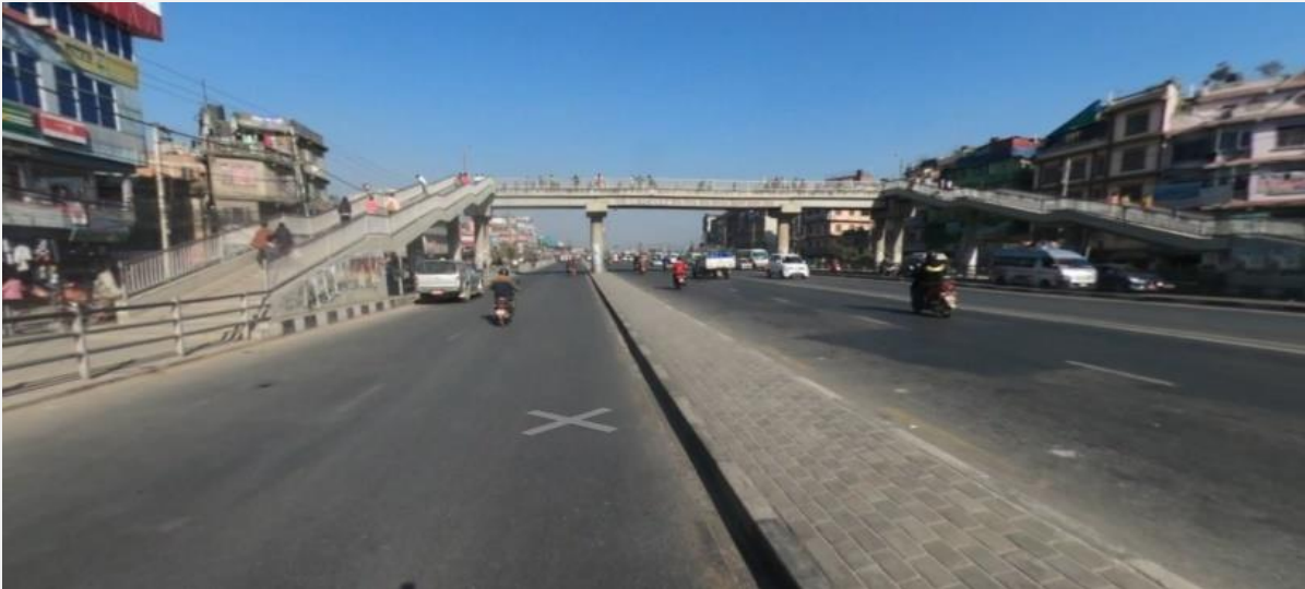
Figure 8: Pedestrian footbridge at Koteshwor, Kathmandu (Source: Googlemap, 2023)
