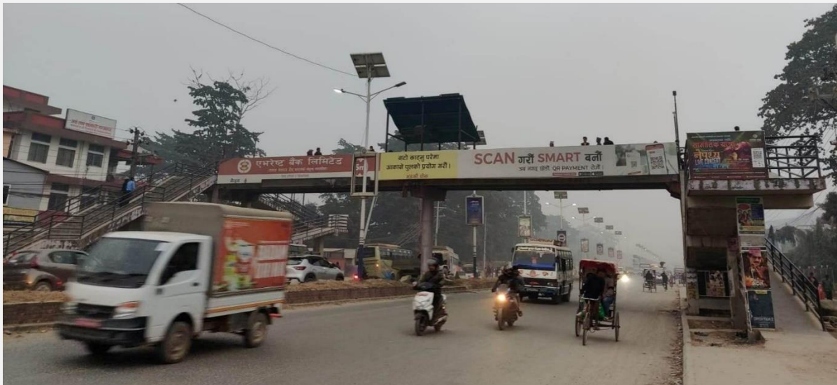
Figure 10: Pedestrian footbridge with ramp in Butwal over Siddharth Highway
