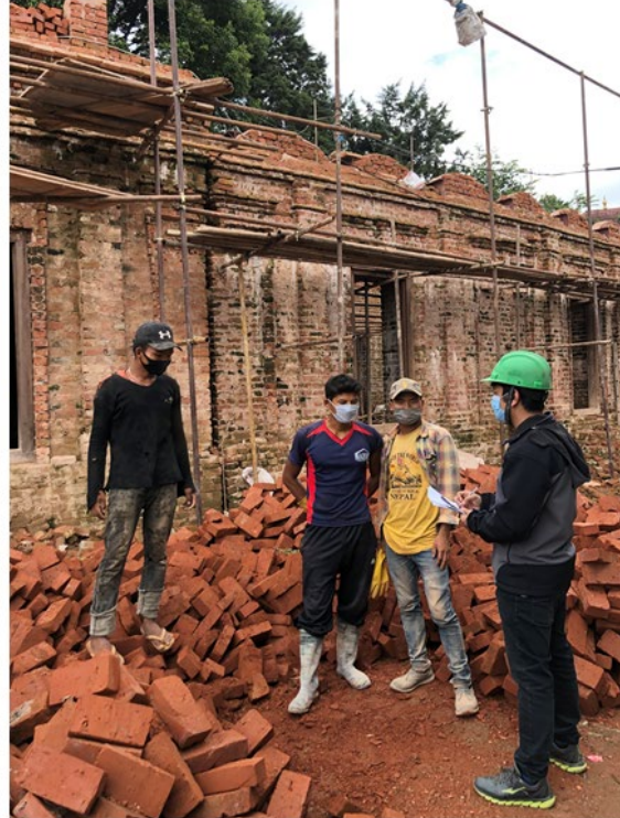
Picture 3: Adjoining building at North and South sides of Singhadurbar West Gate
