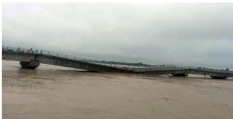
Figure 2: Bridge failure (Jha and Chaudary 2021)
