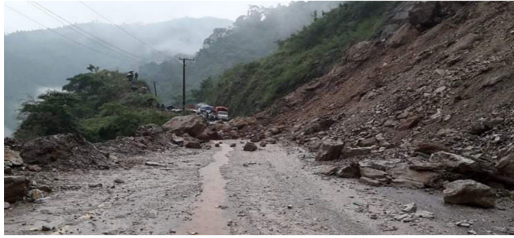
Figure 1: Blocked the Narayangarh-Muglin road section due to landslide 2021 (My Republica, 2021)
