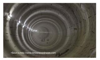
*Figure 9(a) Segmental lining tunnel*
